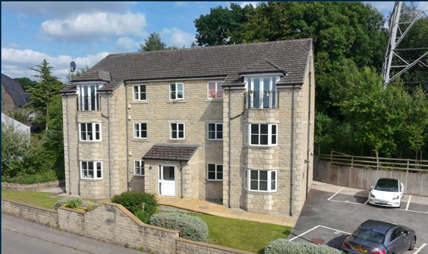
Apartment 6, Pennine House, 18 Barnsley Road, Scisset, HD8 9GJ
